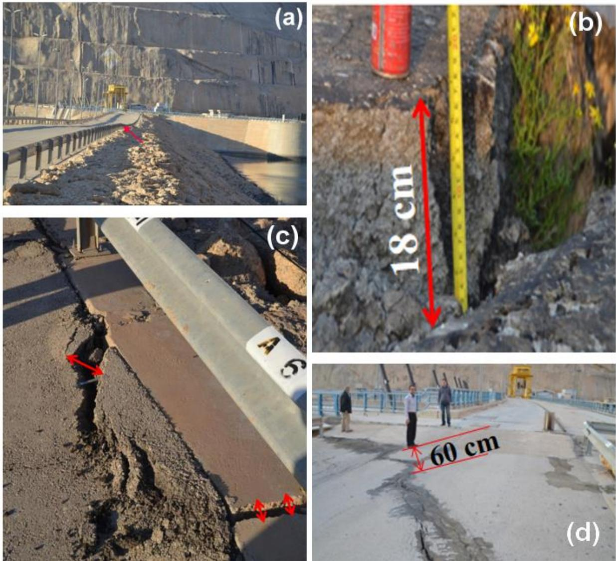
Figure 2. Exemplary ground pictures of damages and cracks of the Masjed-Soleyman dam. (a) Settlement of crest and creep of the upstream embankment, (b) cross cracks along the crest, (c) longitudinal cracks of the crest, (d) vertical displacement and cracks at the crest as a result of the settlement of earth body of dam with respect to the concrete spillway.
