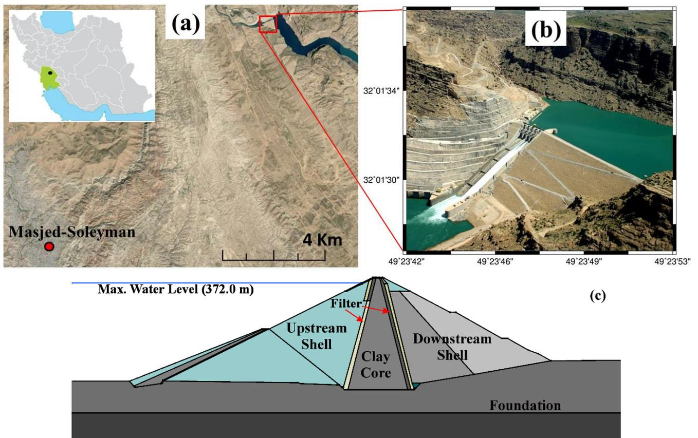
Figure 1. The Masjed-Soleyman dam; (a) Location of the dam in the Khuzestan province, Southwest of Iran; The black circle shows the location of the dam; (b) Embankment, spillway, and the water reservoir of the dam; (c) Cross-section of the dam at the chainage of 260 m including foundation, clay core, filters, upstream and downstream shells.
